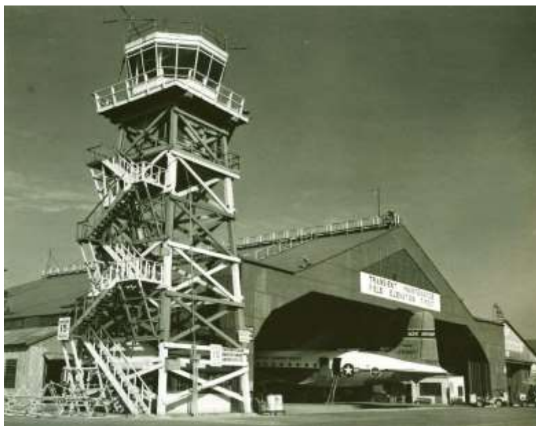
Haneda Air Base Air Traffic Control Tower
